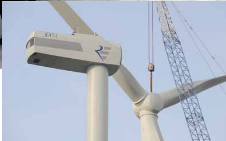
Erection of an offshore wind turbine
